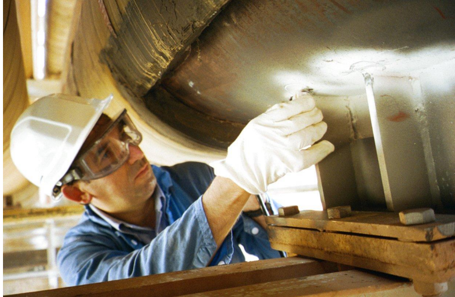
ACFM Inspection of high temperature component using standard probe
