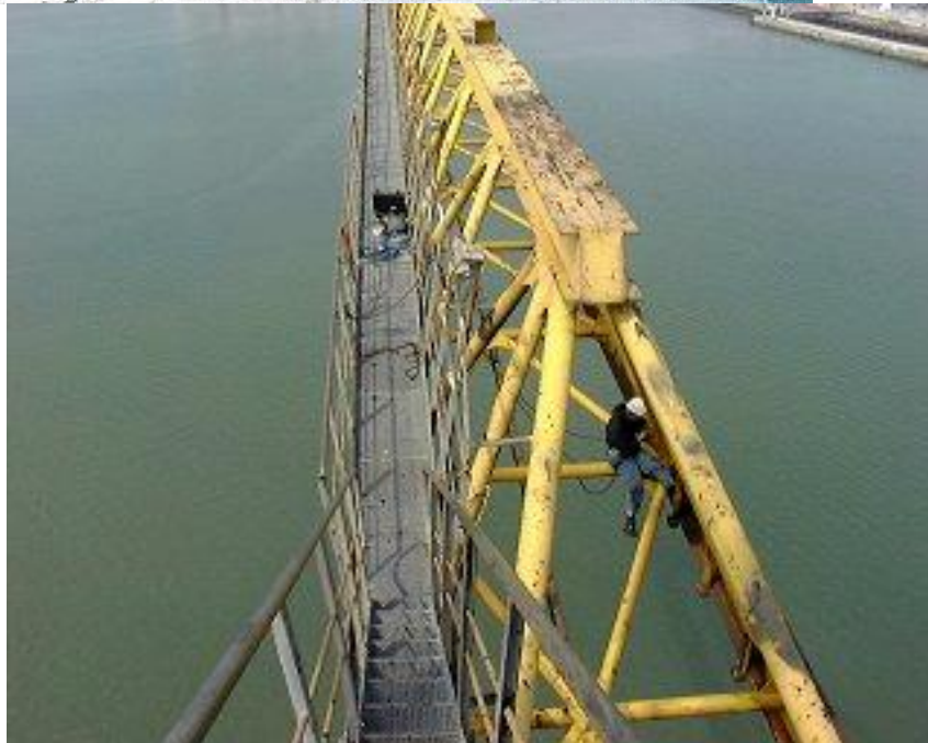
ACFM Inspection by Rope Access
