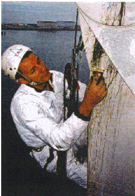
Figure 3. Abseiler inspecting crane
