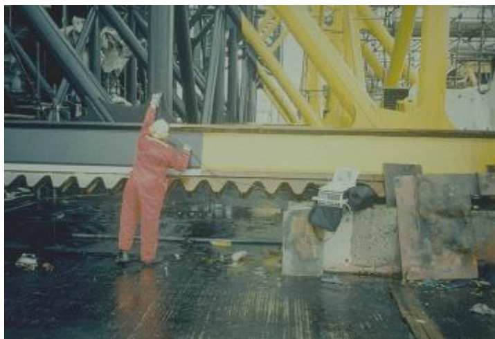
Figure 2. ACFM Inspection of painted jack-up leg
